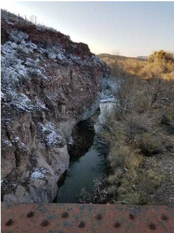
Railroad Trestle over Alamito Creek near fault scarp
